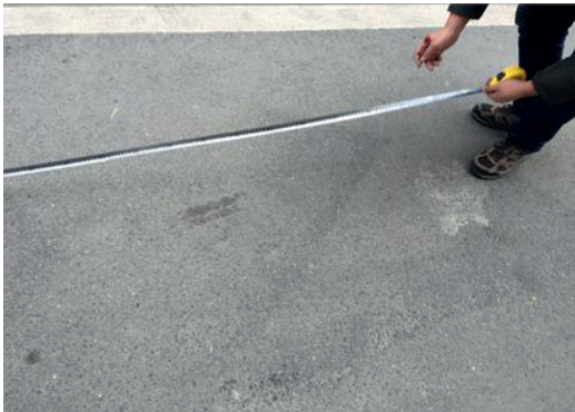
1. Measure the installation position of the geomagnetic field
